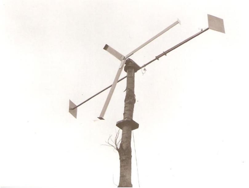
fig. 10 The DRIEKA-4 windmill with double vane and tree tower designed in about 1985
