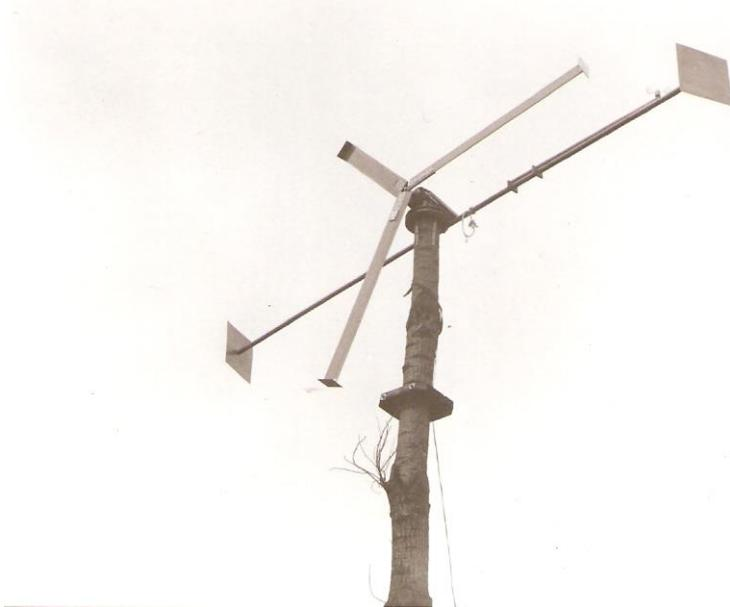
fig. 11 DRIEKA-4 windmill with double vane and tree tower designed in about 1985
